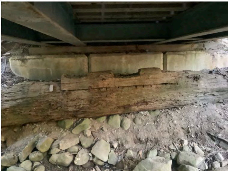
Right Bank Abutment when facing downstream
