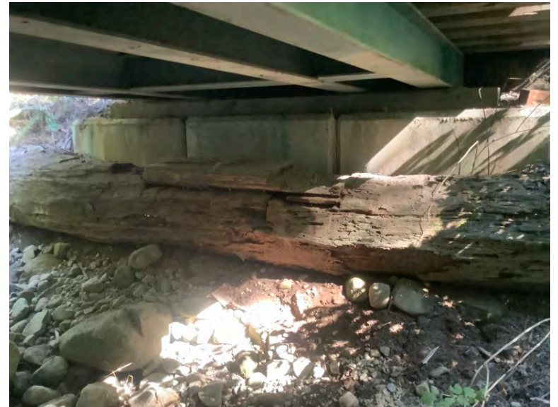
Left Bank Abutment when facing downstream
